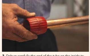
2. Deburr carefully the end of the tube on the inside to minimize turbulence and pressure loss according to AS3500 and on the outside to avoid damaging the O-ring.
