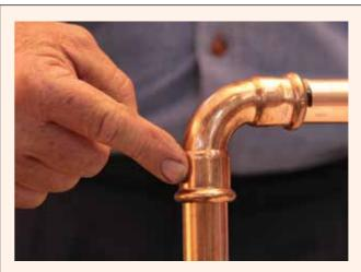
**9.** Visually inspect the fitting to ensure the press has been completed. The KemPress® tool will flash if the fitting did not press correctly. If this occurs a new fitting and tube section is required. At the end of the project visually inspect each fitting to ensure none have been missed.
