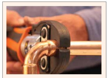
**8.** Initiate the pressing job by pressing the start button. The automatic pressing process guarantees a tight connection. The pressing process can be interrupted by pressing the emergency-stop button.
