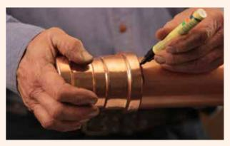
**4.** Mark the insertion depth on the tube by lining up the fitting side by side with the tube or by inserting the fitting onto the tube until it reaches the tube stop. When fitting is inserted onto the tube the outer edge of the fitting must line up with the marking. Refer to the table below for the minimum insertion depth.
