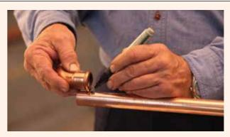
**4.** Mark the insertion depth by lining up the fitting side by side with the tube and mark the tube. When the fitting is inserted onto the tube the outer edge of the fitting must line up with the marking. For correct insertion depths see column e of the Fittings Space Requirements table, page 20.
